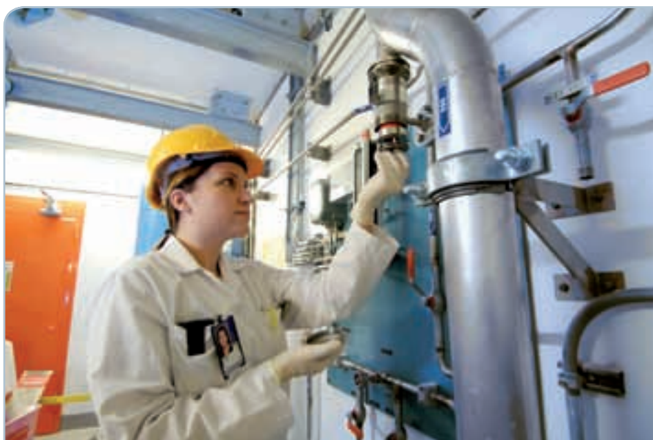
The air flow in the ventilation stack is sampled and measured for the rates of radioactive releases into the atmosphere.
