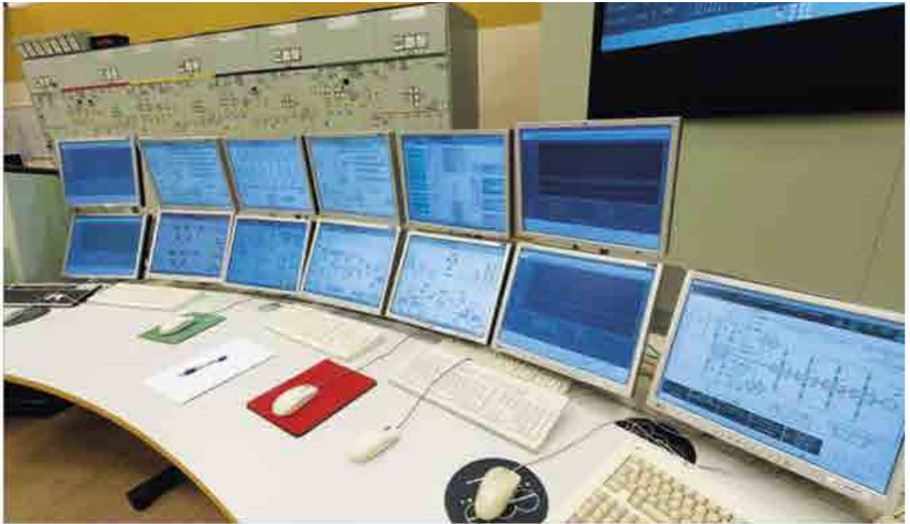
The turbine automation control and display workstations
