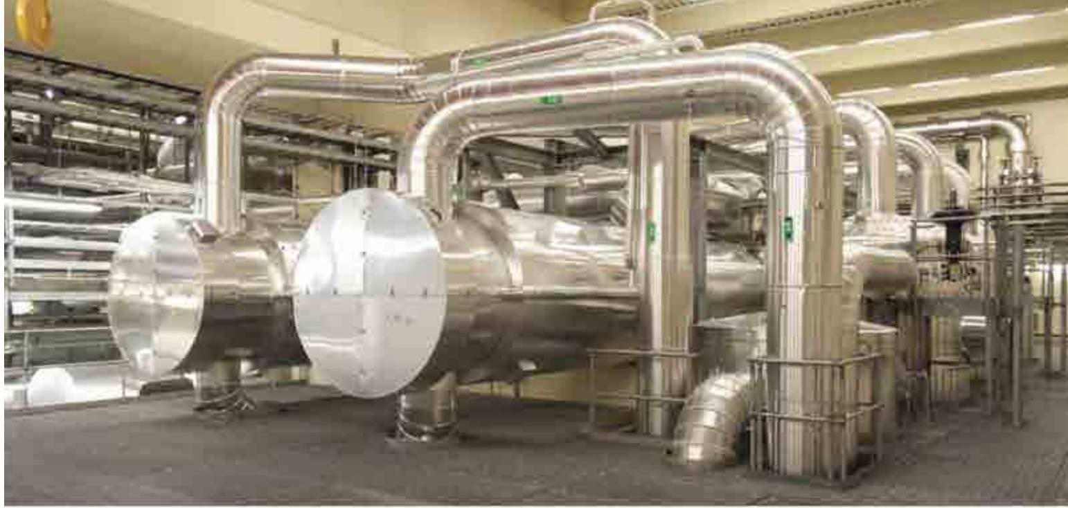
Low pressure preheaters.
