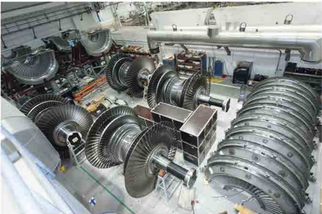
The OL1 and OL2 turbine plants were modernized in the course of the annual outages of 2010-2012. The modernization included, for example, the replacement of the I.P. turbines and the generators.
