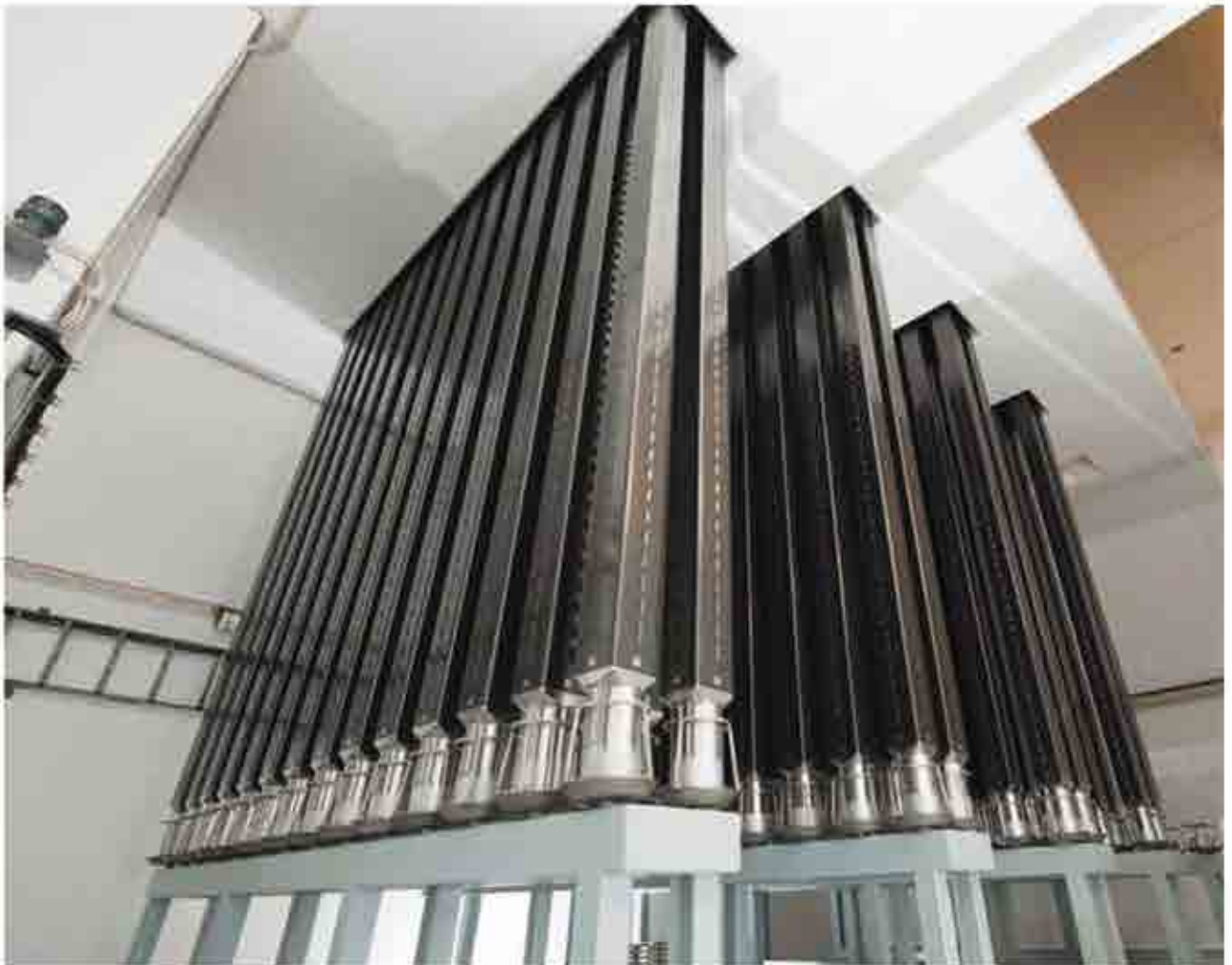
Fresh fuel is stored in the dry storage facilities.
