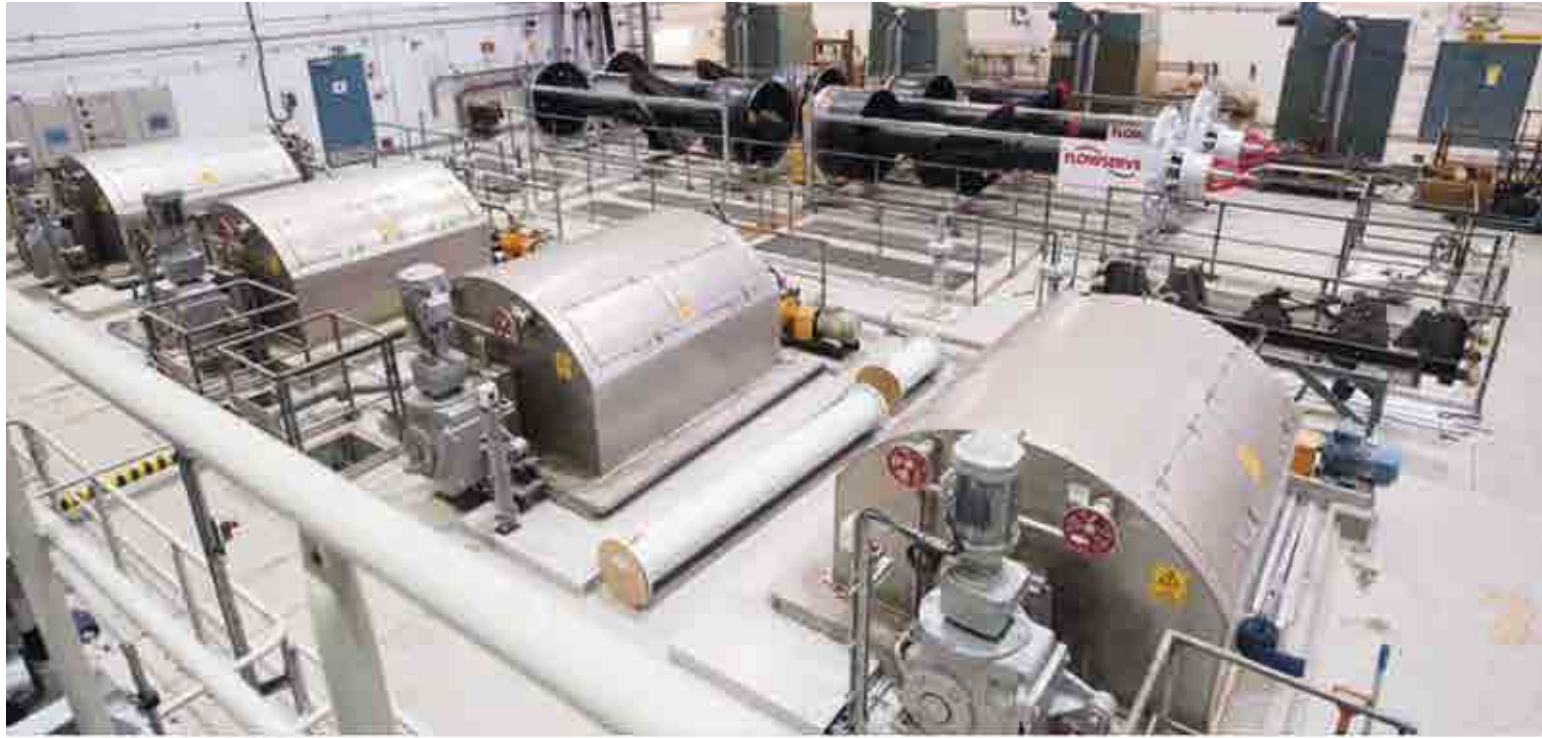
Screening and pumping building
