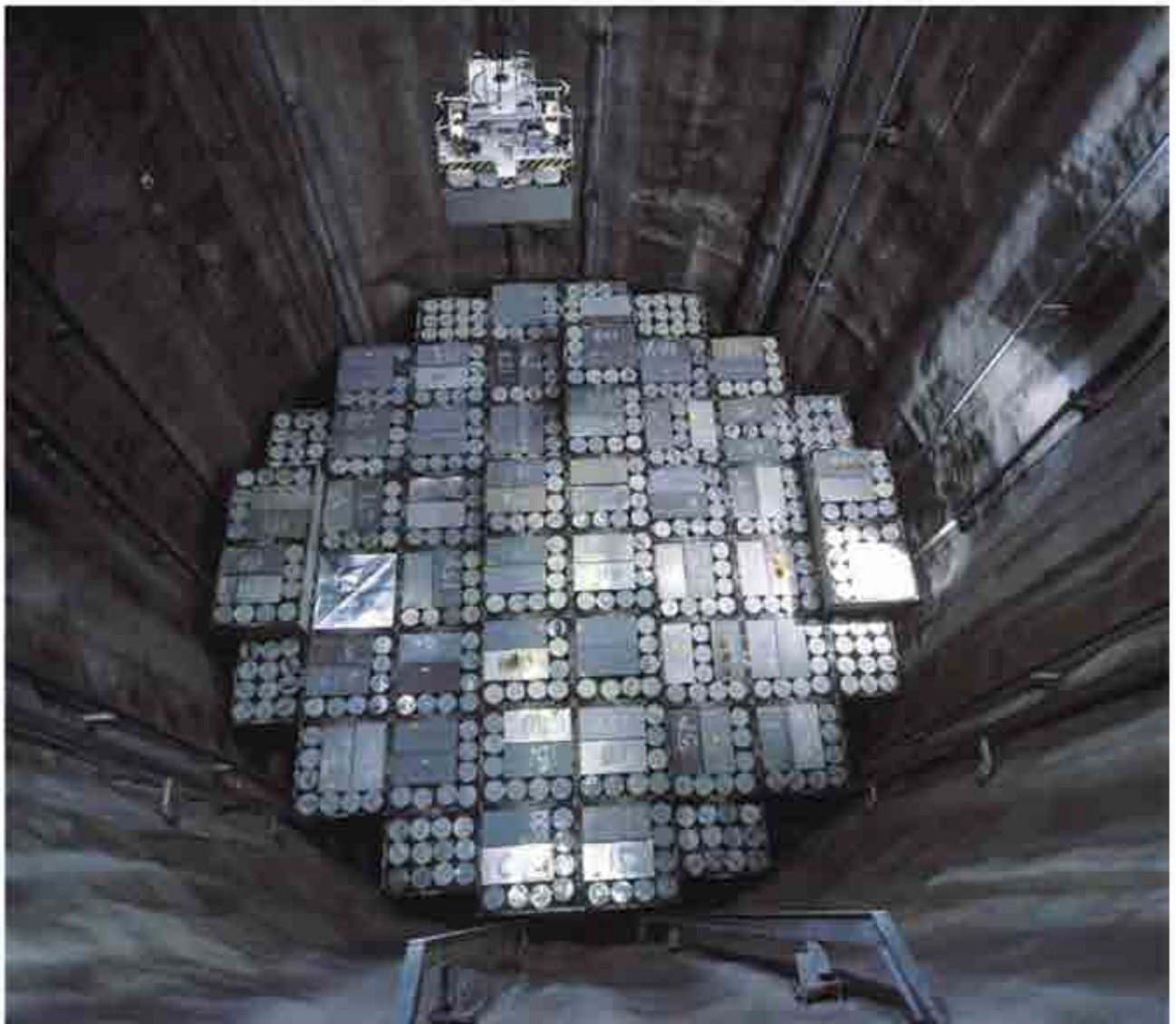
In the operating waste repository (VLJ repository), the concrete containers are transferred into the low level waste (MA) and intermediate level waste (IA) silos, excavated to the depth of 60-100 meters into the bedrock.
