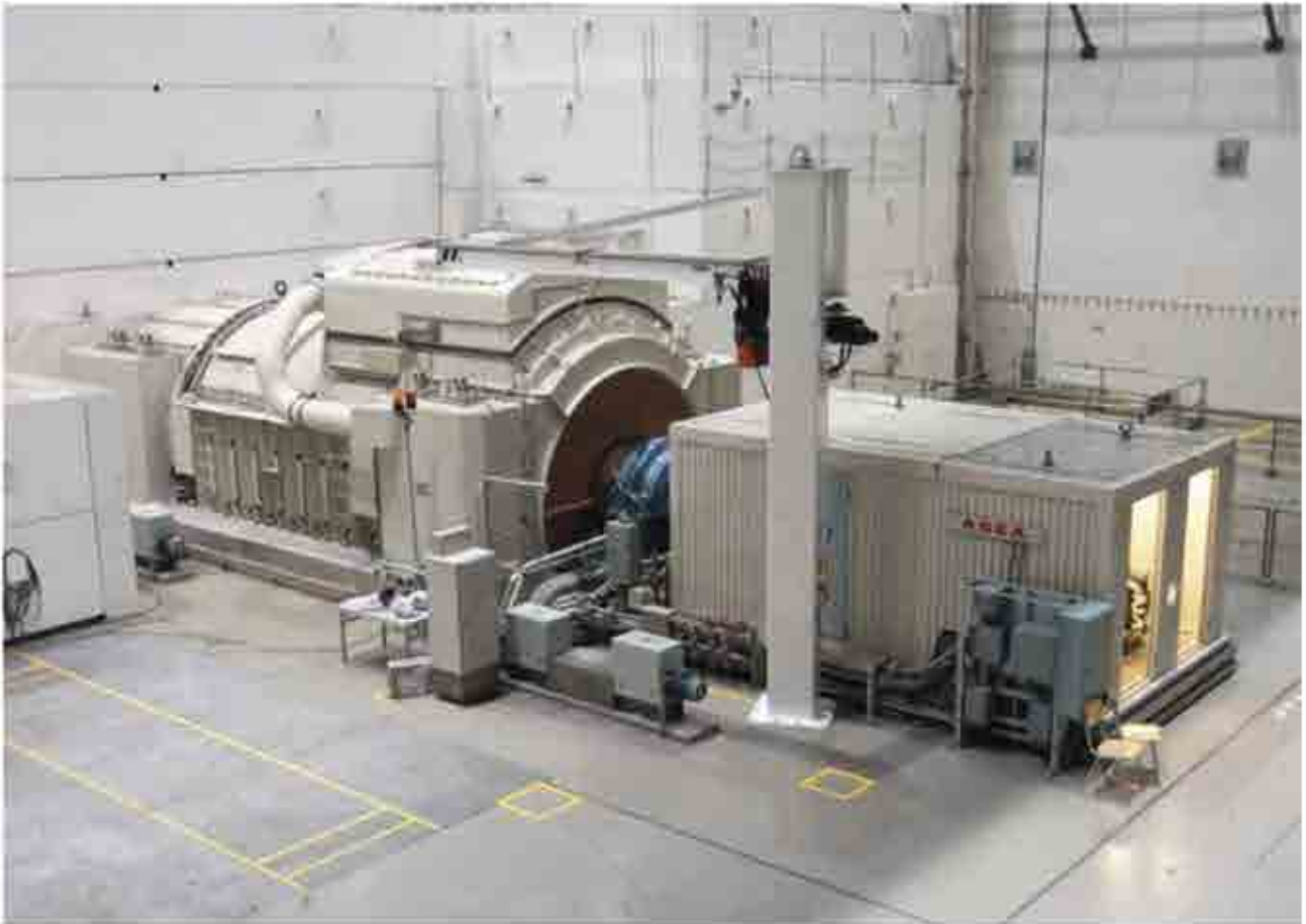
Generator and exciter
