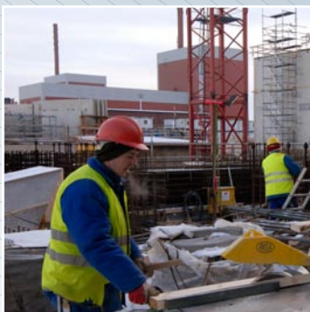
The construction work of the OL3 project continued all year.
