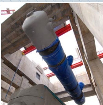
The equipment installations were started in OL3's turbine building.
