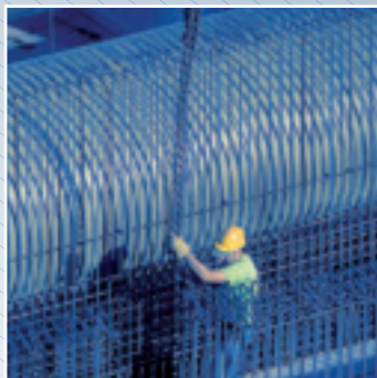
Installation of sea water pipes proceeded at the OL3 site.
