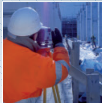
Construction at the OL3 turbine plant proceeded.
