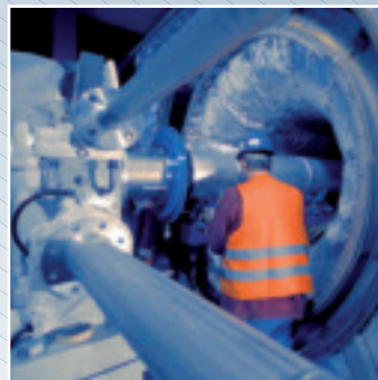
Construction and installation work at the gas turbine plant.
