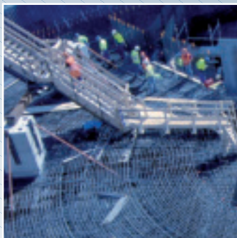
Concrete reinforcement work at the OL3 reactor building.
