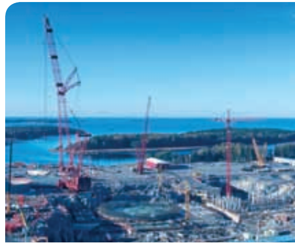
The OL3 foundation was mainly carried out by Finnish employees.
